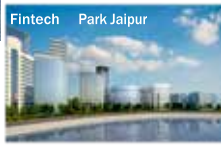
Plug And Play Facility At SEZ, Jaipur
